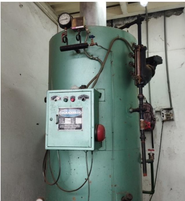
Figure 1. Boiler of the animal processing plant.
